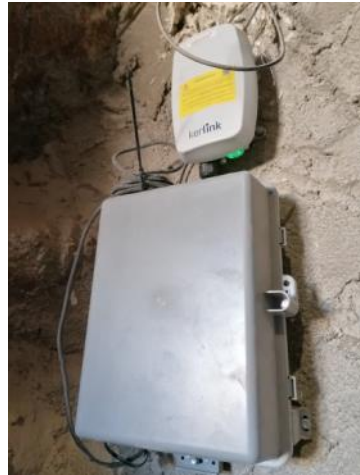
Gateways (LoRa system)
